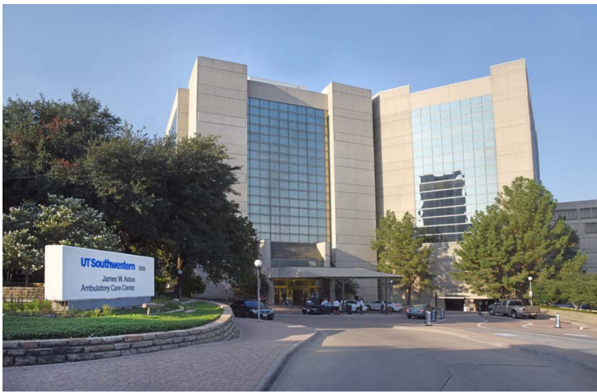
The James W. Aston Ambulatory Care Center has been undergoing renovation to optimize and add space for clinical research.
