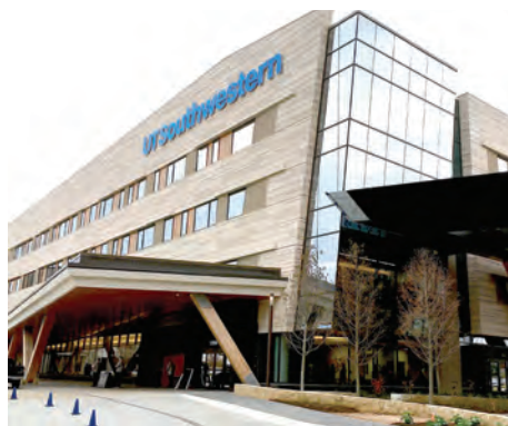
On Dec. 3, UT Southwestern Frisco opened its doors to clinical care in a new 120,000-square-foot, state-of-the-art medical building.
